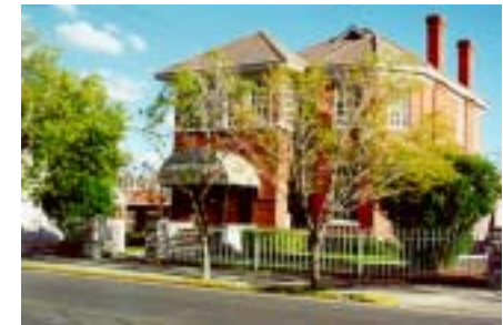
Office with screened parking in the rear.
