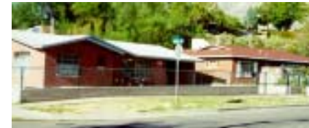
Chain-link fencing is prohibited.
