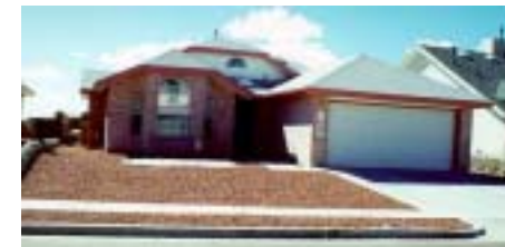
Graveled yard without appropriate vegetation.
