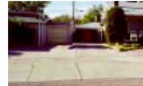
Inappropriate abutting driveways without a landscape buffer.
