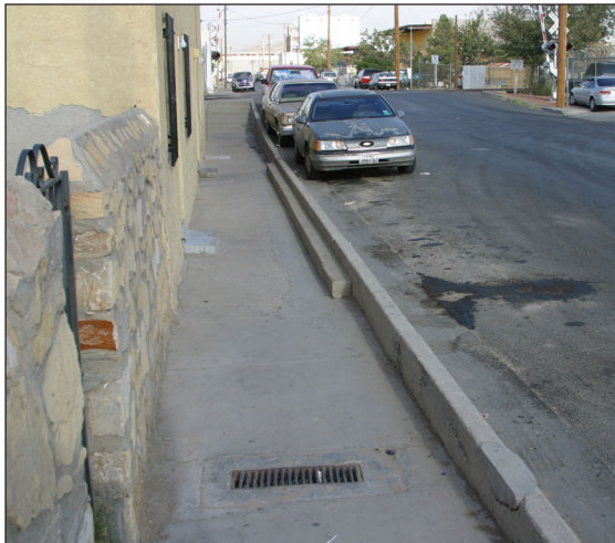
Above: This high curb on Canal St. attempts to divert floodwaters away from the residence and into a nearby culvert intake in the street. The sidewalk is drained during storms by its own small intake.
